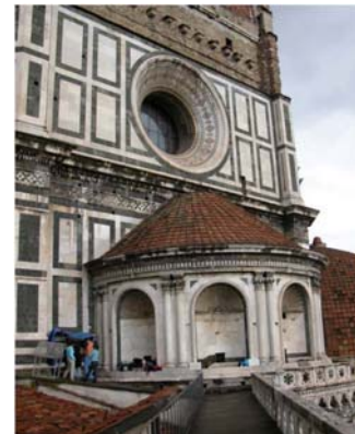
Figure 4. In situ test area.
