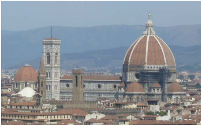
Figure 3. Florence Cathedral. View from south.
